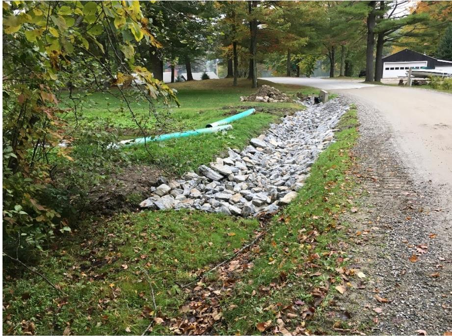
**Third and final run of ditch line rehabilitation completed by Mitchell Excavating.**
