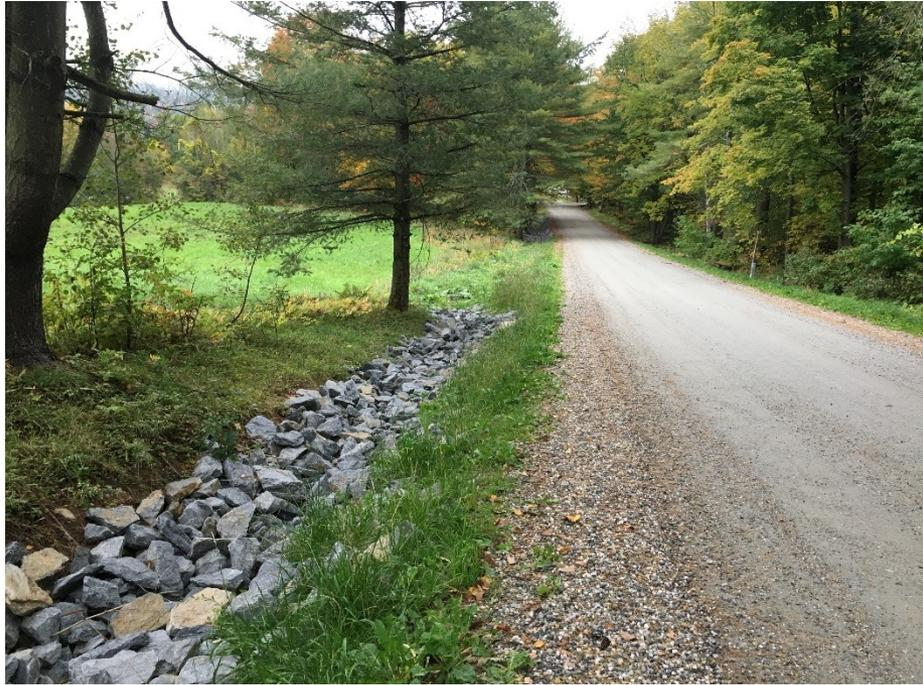
**The first 650 feet of rehabilitated ditch line ends with a turnout.**
