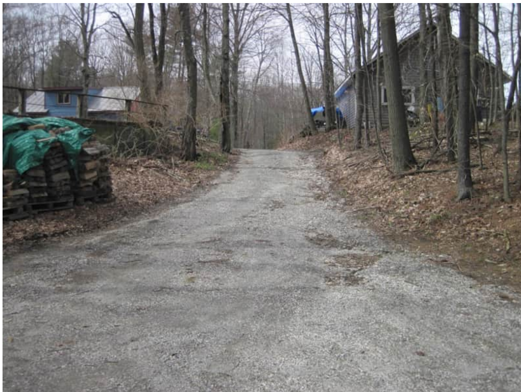
Figure 34: Project 28 – Southwest Shore Road improvements
