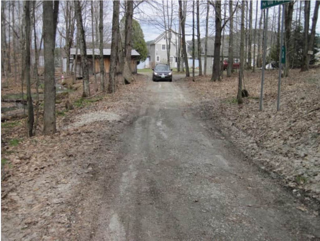
Figure 35: Project 29 – Old Pump Road improvements
