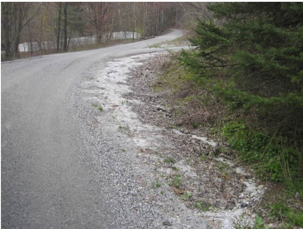
Figure 26: Project 23 – Kozas Run improvements
