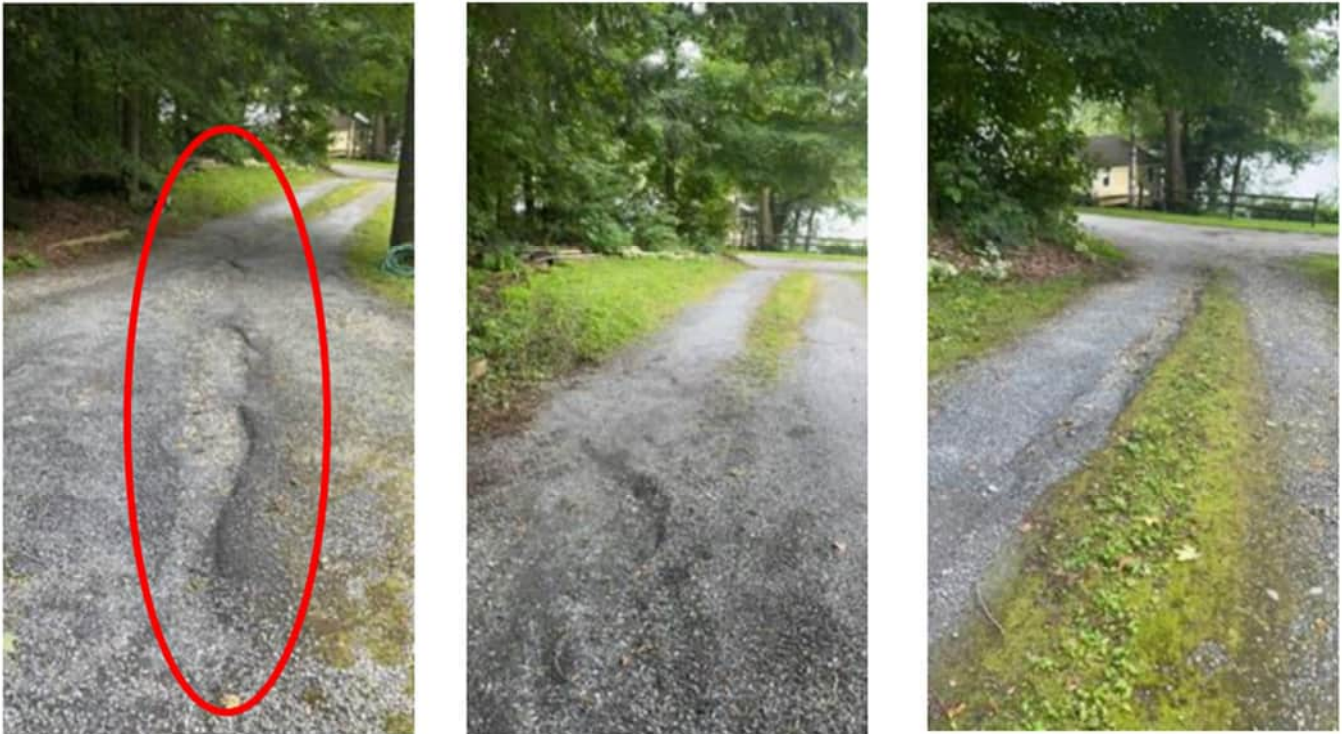
Figure 65: Project 58 – Driveway improvements at 56 Dimick Road (photos from WNRCD)
