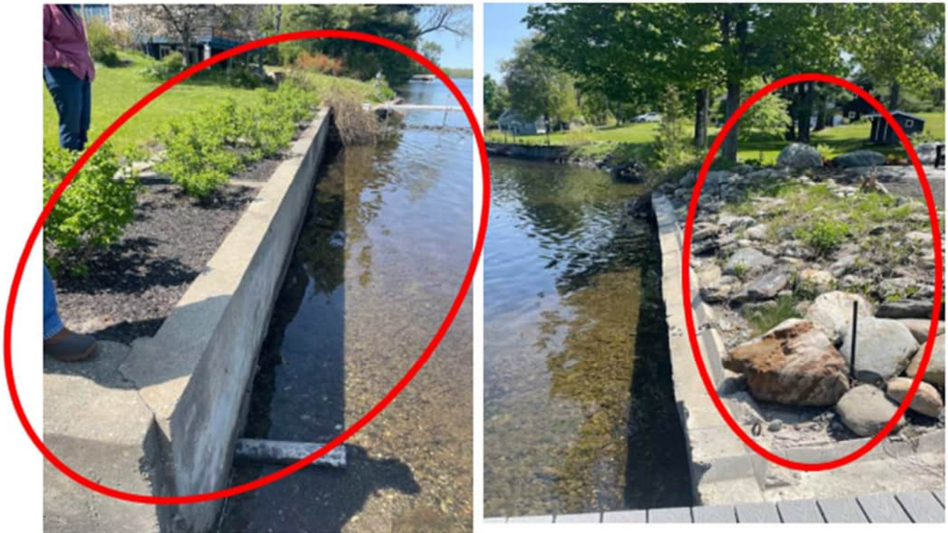
Figure 14: Project 12 – Sea wall removal and bank restoration along Pine Shore Drive (photo from WNRCD)
