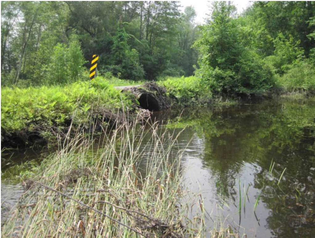
Figure 15: Project 13 – culvert replacement at Beebe Lane
