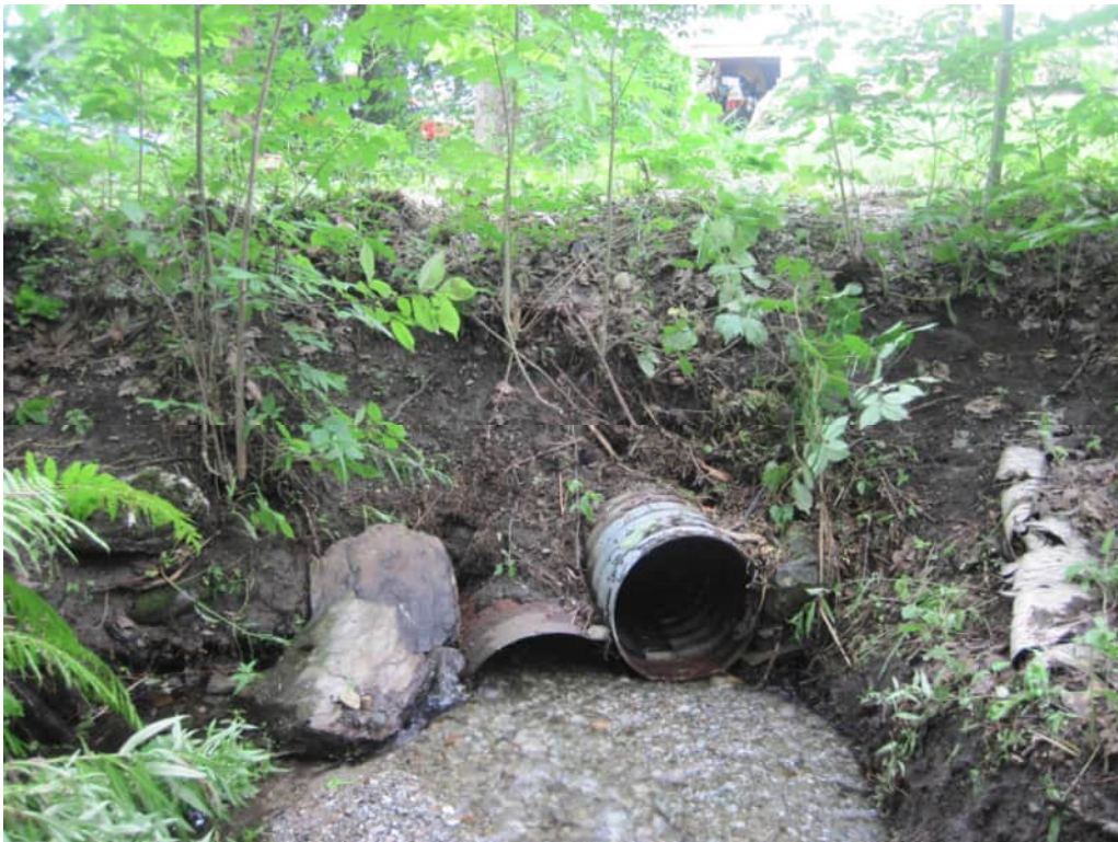
Figure 20: Project 19 – culvert replacement on Old Pump Road
