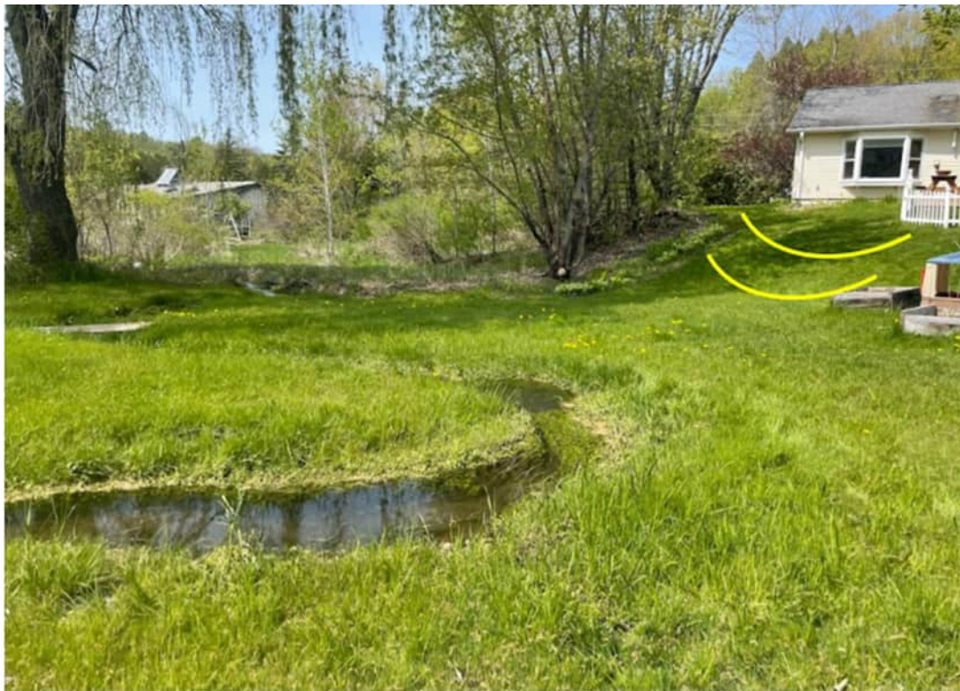
Figure 62: Project 55 – Filter berms at 114 Hawk Lane (photo from WNRCD)
