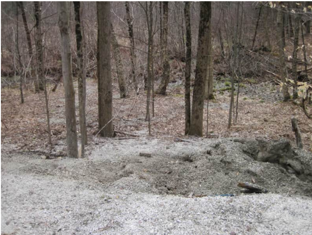
Figure 32: Project 26 – Pikes Point Road improvements
