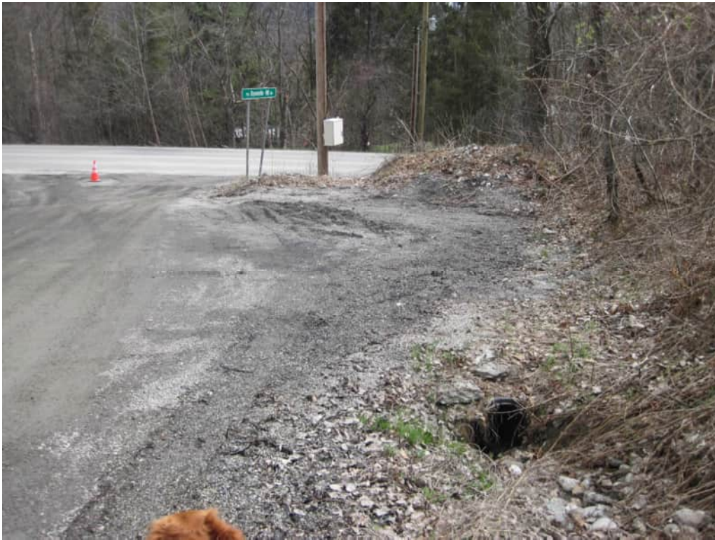
Figure 25: Project 22 – Dynamite Hill Road improvements
