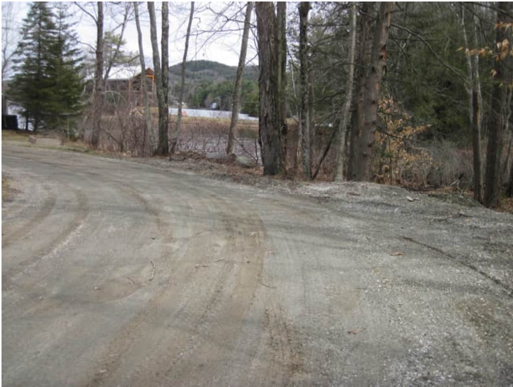
Figure 31: Project 26 – Pikes Point Road improvements
