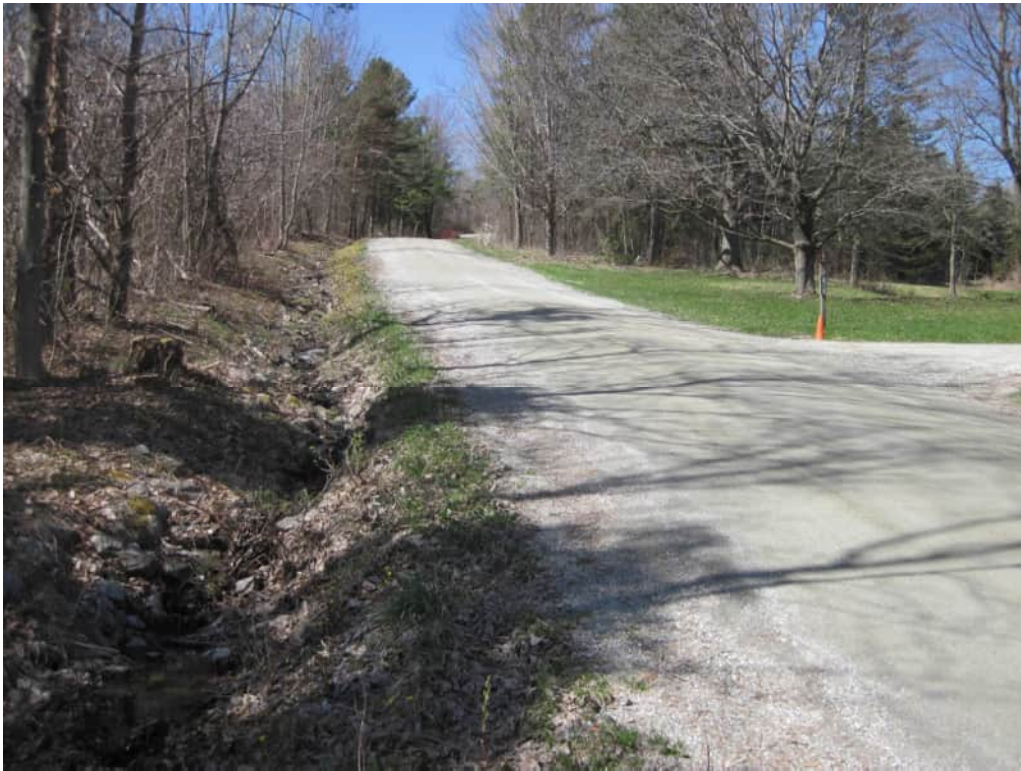
Figure 23: Project 21 – Mount Pritchard Lane improvements
