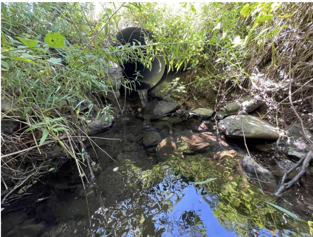
Figure 2: Project 2 – culvert replacement at Richmond Road
