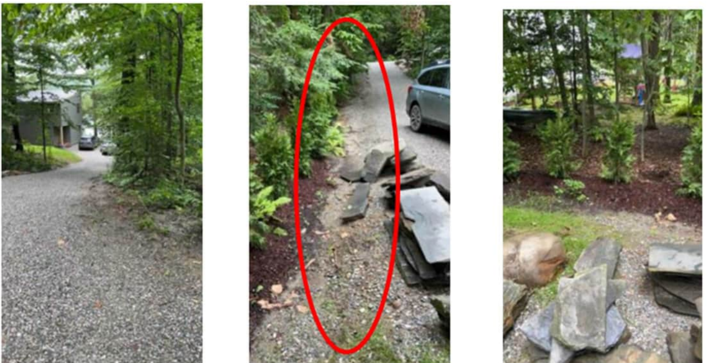
Figure 64: Project 57 – Driveway improvement at 840 Beebe Lane (photos from WNRCD)
