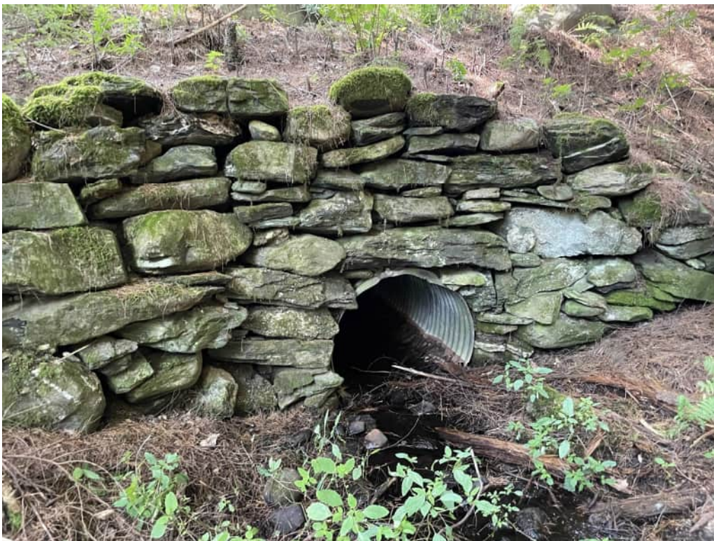
Figure 6: Project 6 – culvert replacement at Hidden Pasture Lane
