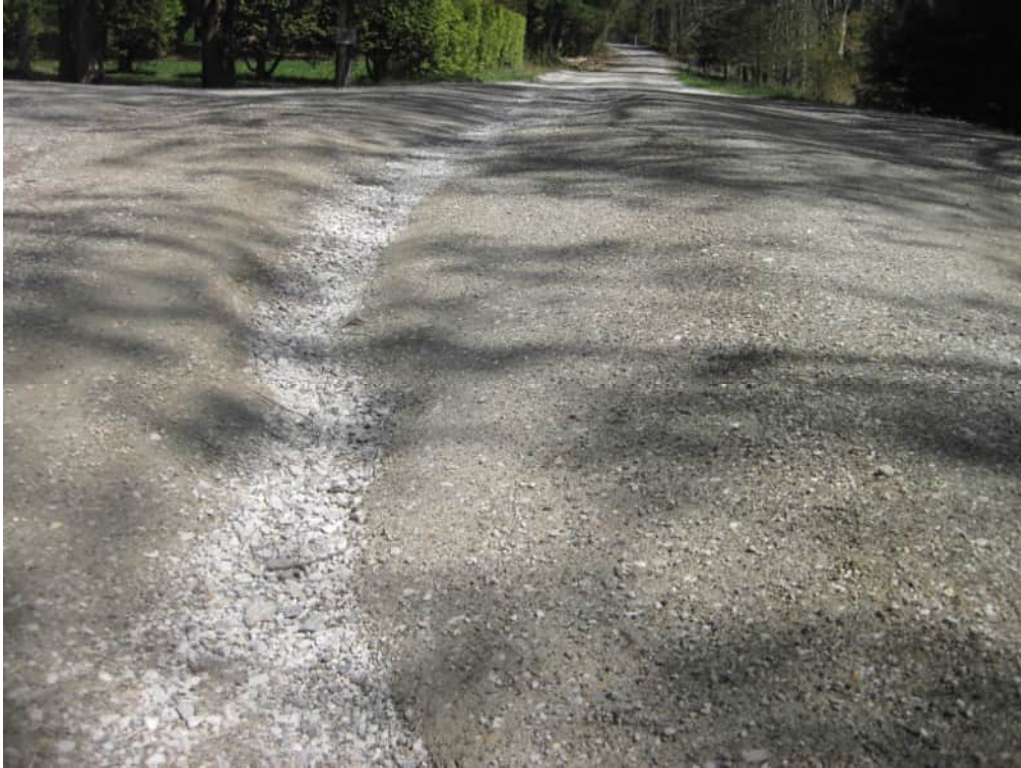
Figure 51: Project 44 – Partridge Hill improvements
