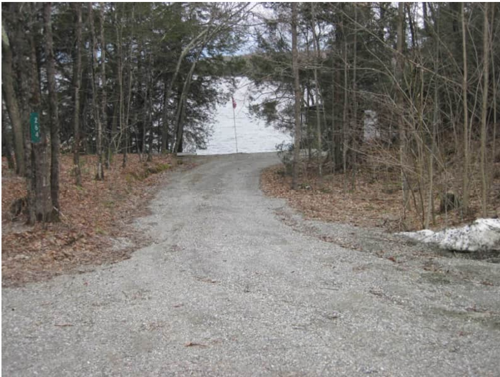
Figure 36: Project 30 – Upper Access Road improvements
