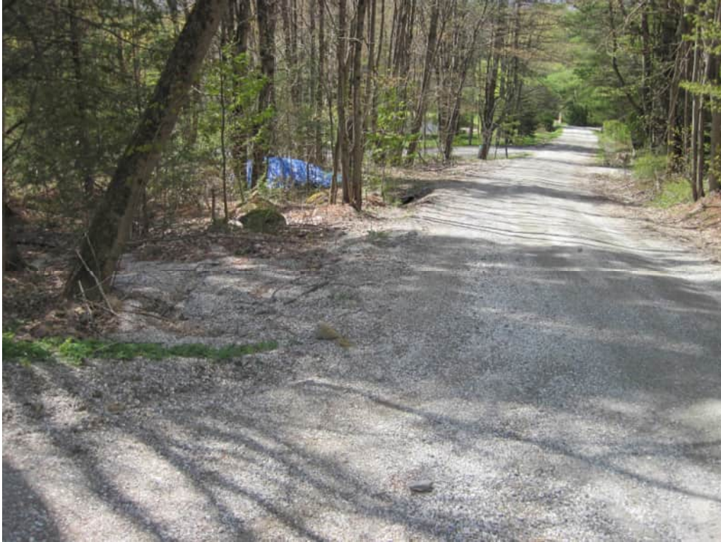
Figure 49: Project 44 – Partridge Hill improvements
